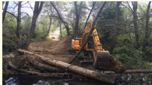
A historic levee is breached along Scotts Creek to increase connectivity between the channel and the floodplain. This project supports floodwater storage, fisheries, and groundwater recharge. Credit: Jim Robins.
