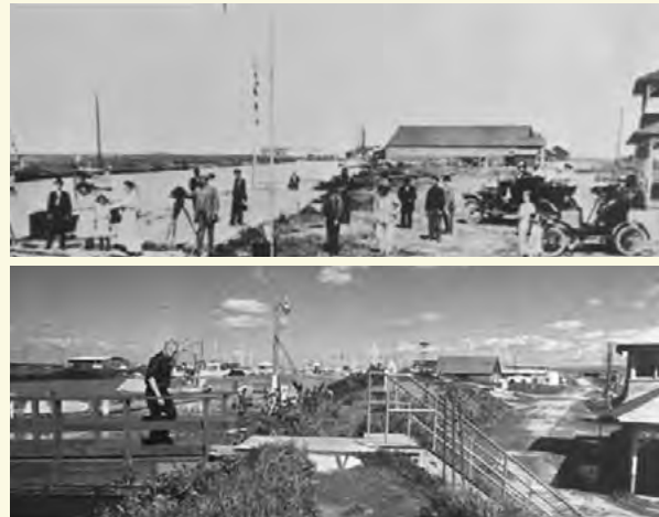
Over decades, groundwater extraction from the Santa Clara Valley aquifer caused land to subside. The top photo shows the South Bay Yacht Club in Alviso sitting near sea level; in the 1978 photo below, the Club sits about 10' below sea level, with a high levee protecting the Bay from flooding Alviso. Credit: Courtesy SCVWD.
